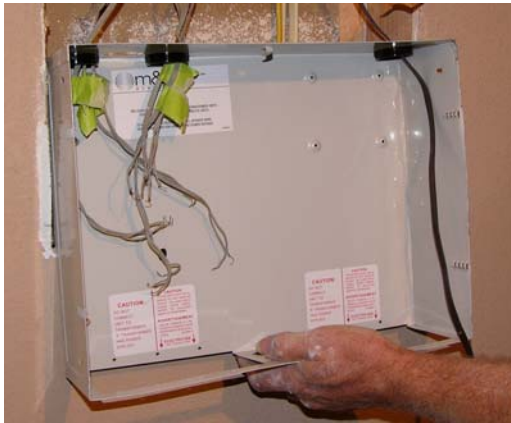
Figure 2 - dmc1H or dmc1HC wall housing placement
