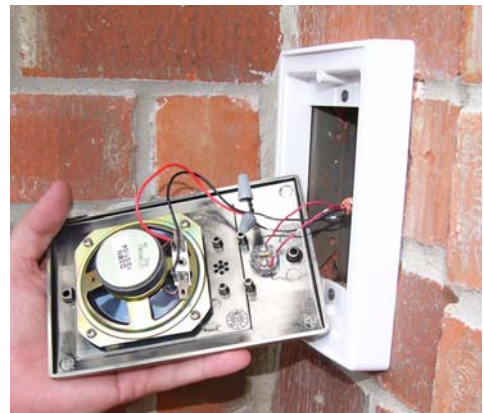
Figure 9 - DMCFD and Door Station Installation
