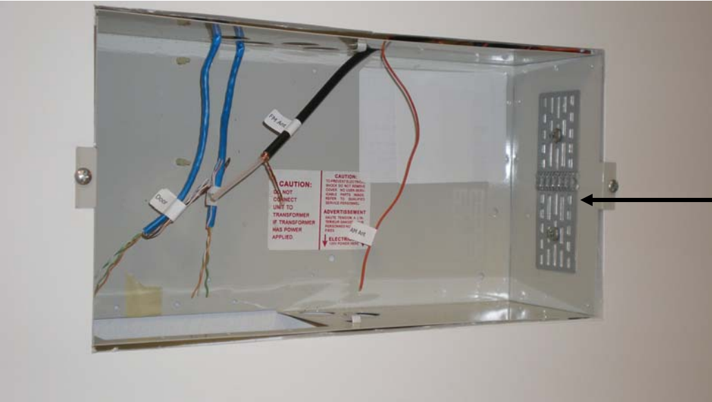
Mounting strap centered between top and bottom of housing. Set back from front edge is 1/2 inch max.
